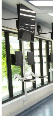
ICWUSA.COM, Inc. can devise mounting solutions for all spaces. In what would usually be considered unusable space, this custom-built "pipe-over-glass" installation shows computer stations mounted in front of windows. These mounts can move both horizontally and vertically,
