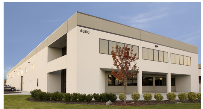
Grumman Building: Assembly and Shipping
