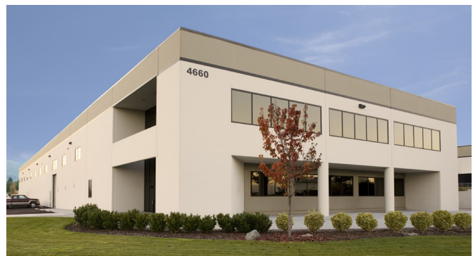
Grumman Building: Assembly and Shipping
